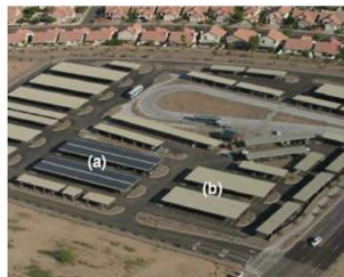
(b) shading with canopy and solar panels [65]
